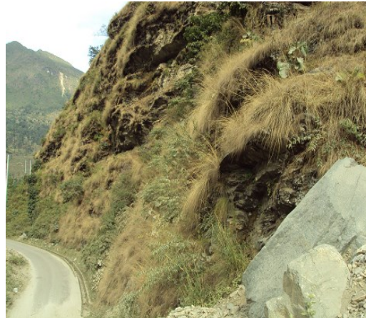
Figure 4: Landslide at specific site (source Subedi, N., 2010)
