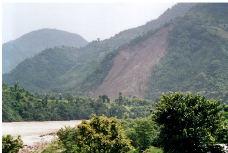
Figure 1: Massive rock slope failure along Prithvi Highway in Nepal
