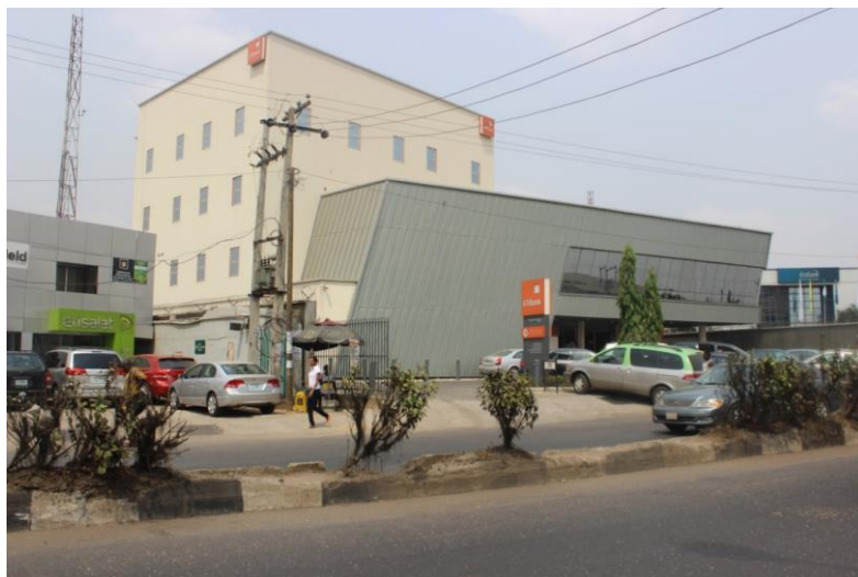
Figure 3: Gtb ogba showing the rheinzink cladding(source: authors photography)
