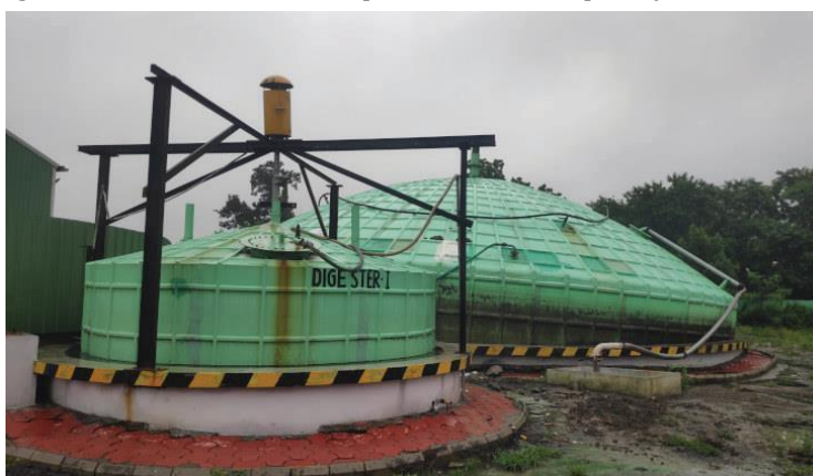
Figure 6: The bio-methanation facility opposite the vegetable and fruit market. Organic waste is converted to fuel used by city buses and as cooking fuel.
