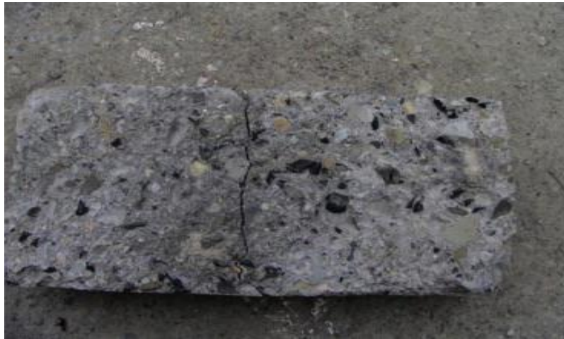
Fig 4: broken concrete samples
