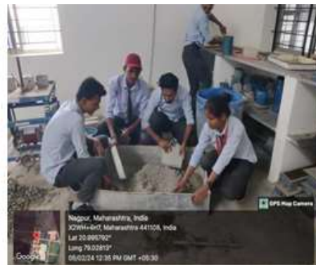
Fig 2: Mixing of materials
