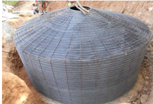
(a) Reinforcement cage for water tank
