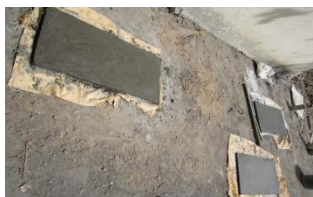
(b) Cement mortar applied to the reinforcement
