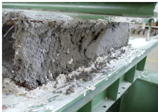
(a) Crushing of web at ultimate load
