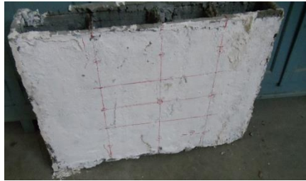
Fig. 14: Mortar applied on weld mesh
