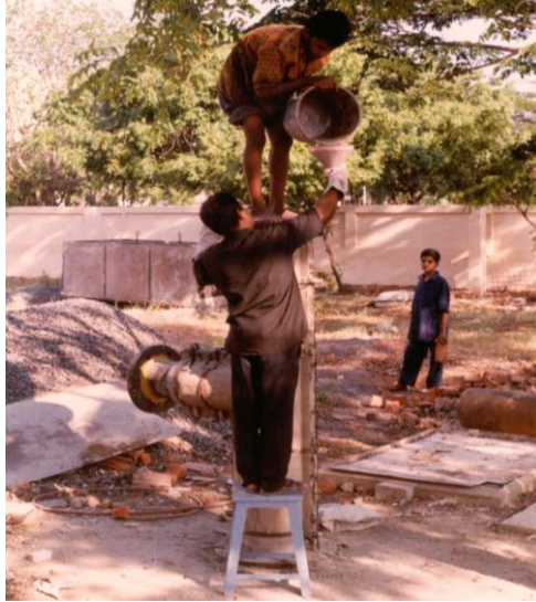
Fig. 9: Pouring of Grout
