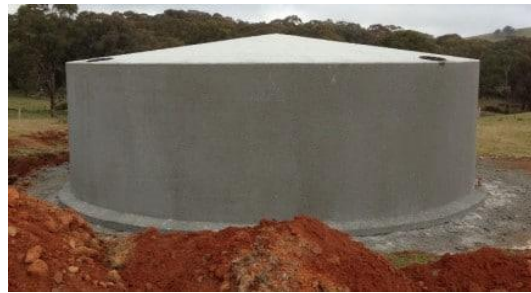
(b) Finished tank
