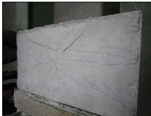
(a) Crack at the Bottom of the Tested Panel
