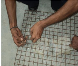
(a) Fabrication of Reinforcement
