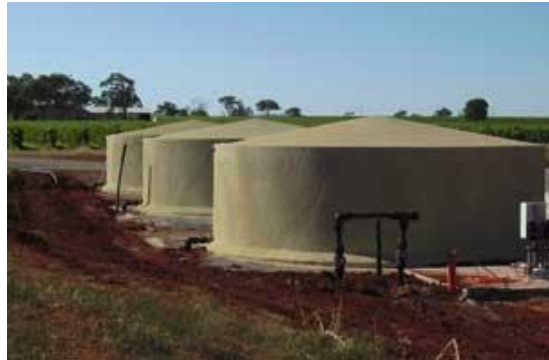
Fig 2: Ferrocement cylindrical water tanks
