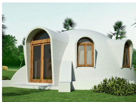
Fig 4: Ferrocement Curved House
