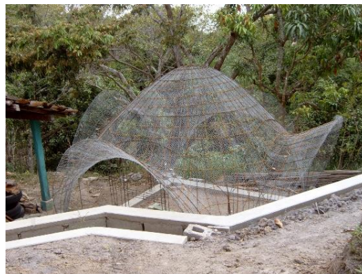
Fig 3: Ferrocement Dome Structure
