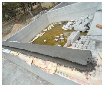
Fig 9: Casting of I Beam and Curing in Pond of Water
