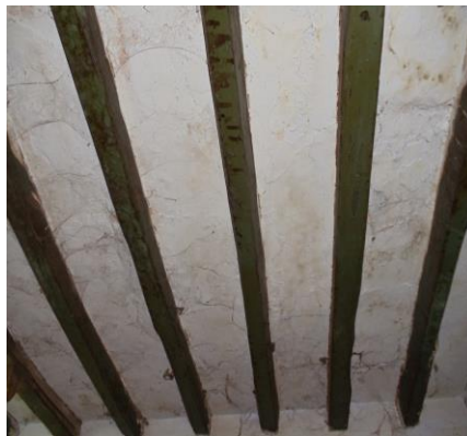
Fig 5: Wooden Reapers, Brick & Lime Mortar Roof in Age Old Building
