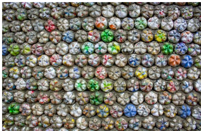
Figure 1: View of eco-brick wall.
