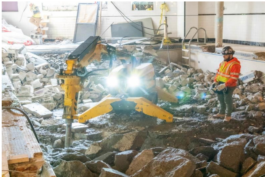
Fig.3 Demolition Robot in India
