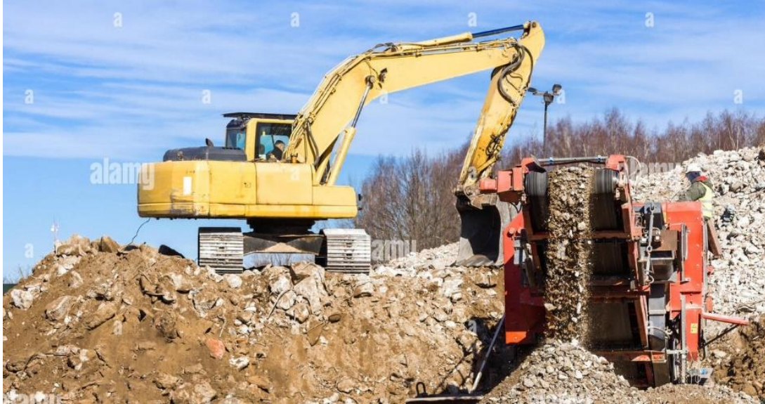
Fig.2 Concrete Crusher Robot in India
