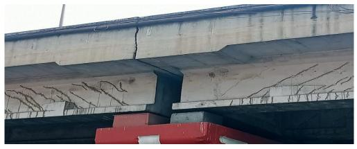
**Fig. no.3** Cracks Developed On Psg Girder At Hadapsar, Pune, Maharashtra Bridge. Due To Excessive Loading And Design Failure.
