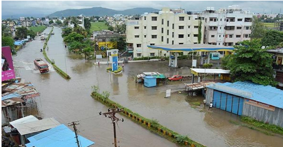
Figure 1: Situation in Pune during flood
