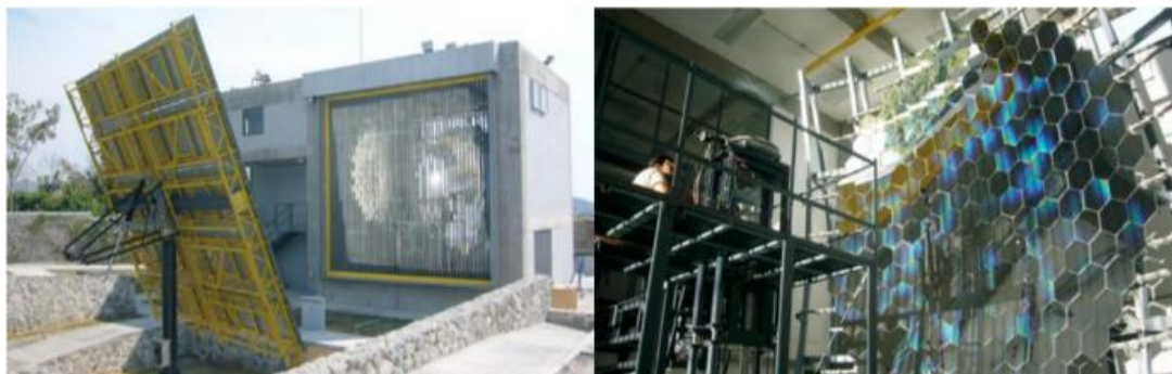
Fig.-5: Showing Heliostat and Shutter on the left and Concentrator on the right [6]
